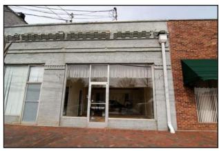
It is important to maintain and preserve the historic roof cornice. Any material that needs to be replaced should be done with materials that match in color, texture, size, and strength. 6966 Main St.
