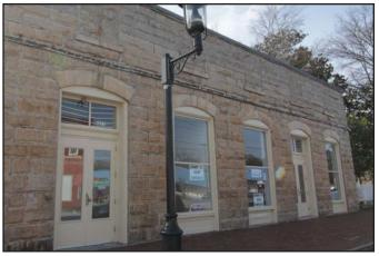
This structure has retained the size and number of historic openings. It is not recommended to enclose or change the size of the door openings. 6957 Main St.
